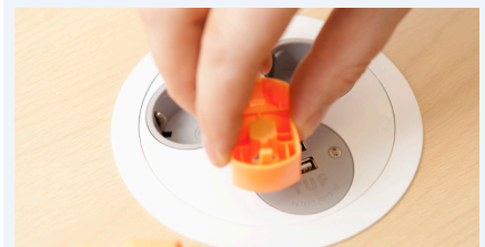
Use the tool to unscrew the 'snake eye' screws.
